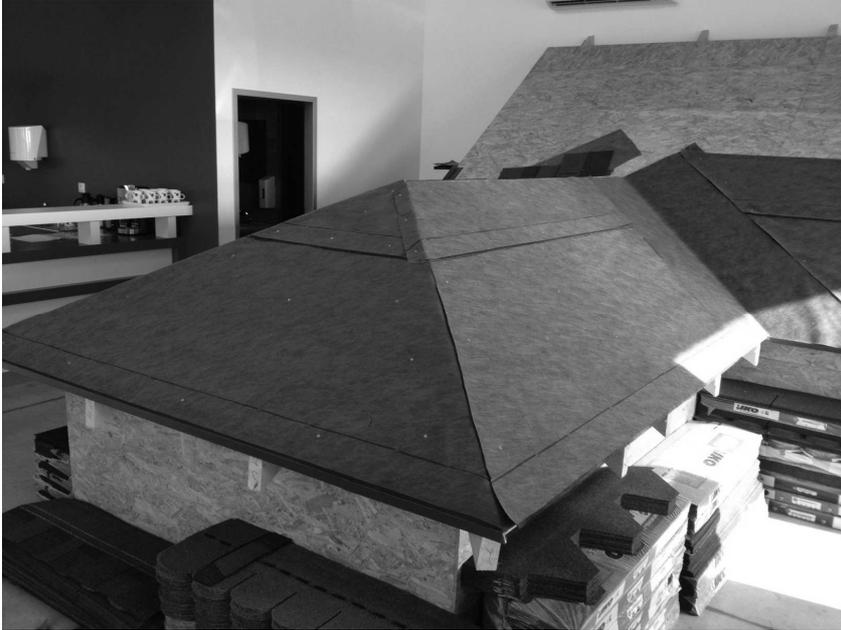
Wood construction with Underlayment for additional safety of the roof.
